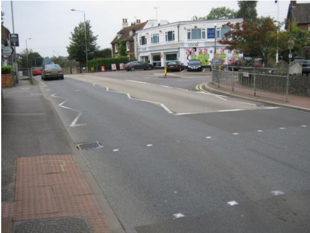
Photograph No.9 – A25 junction with High Street
