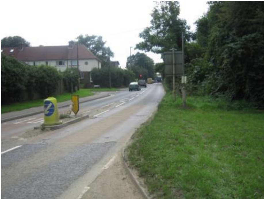
Photograph No.2 – Dilapidated island and activation of VAS (background)
