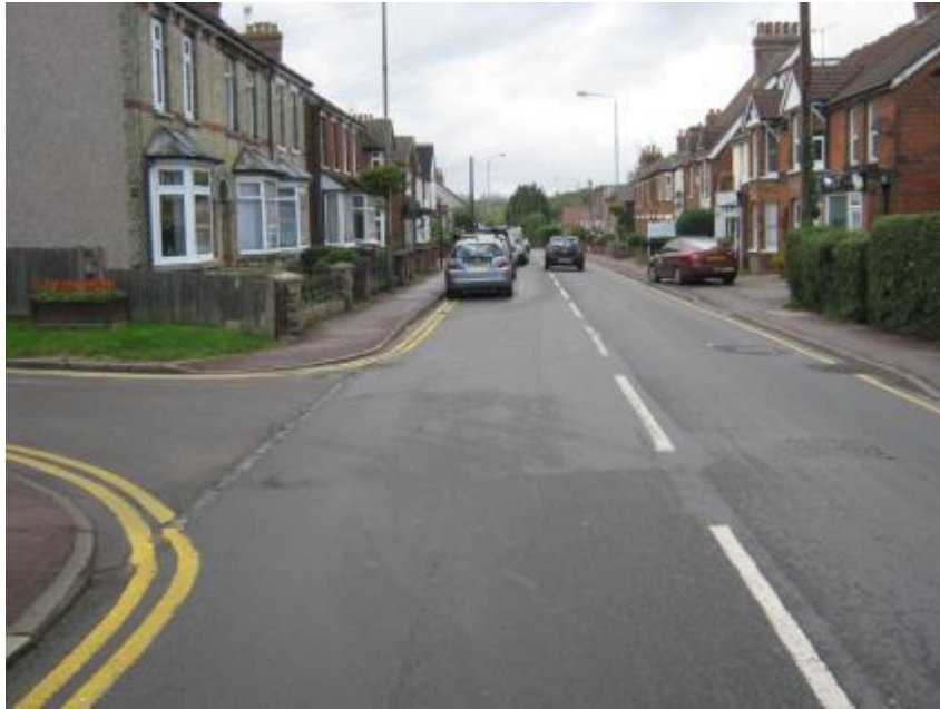
Photograph No 23 – looking west, On-street parking
