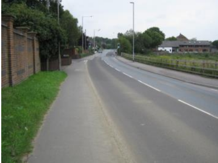
Photograph No.4 – Good standard of road and intermittent frontage development
