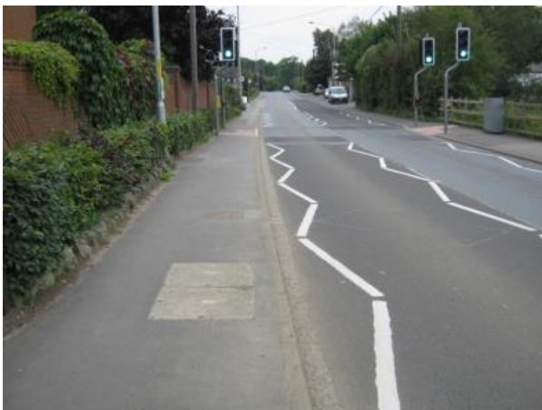
Photograph No.5 – Recently installed signal controlled pedestrian crossing (Puffin)
