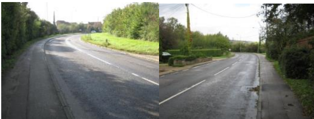
Photograph 17 & 18 – sharp bend at BG landfill site, s/b and n/b respectively
