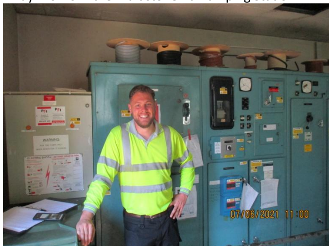
Andy Morris in the Maidstone Rd Pumping Station
