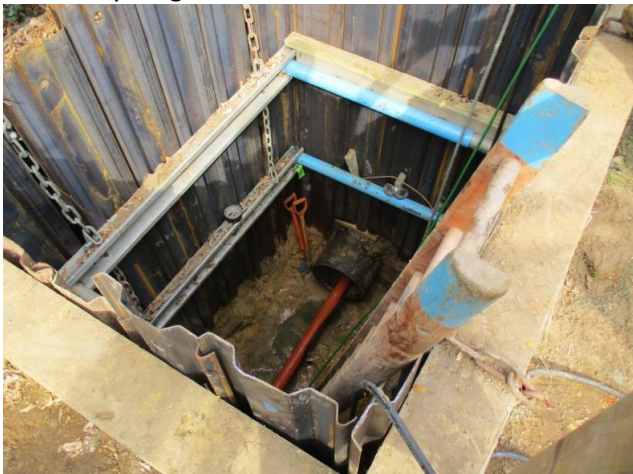
First Sandy Ridge Excavation
