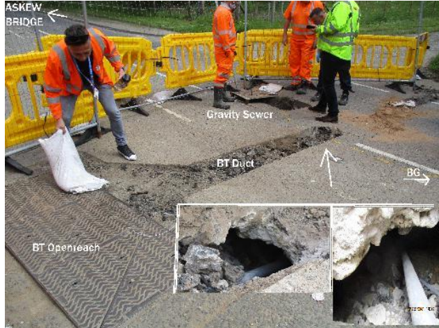
KCC and SW investigate the collapse
