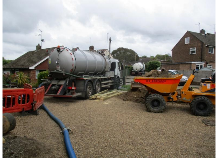
Standby tankers keeping excavations clear
