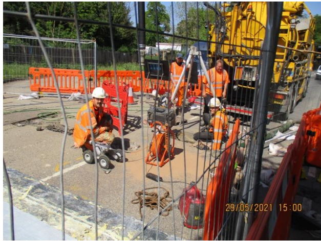
Specialist team CCTV survey the pipe and prepare a Resin Repair
