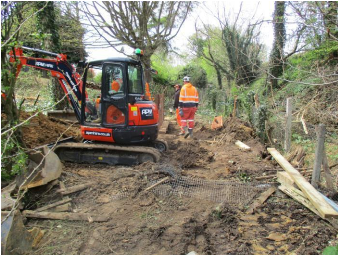
Site of third sewage breakout
