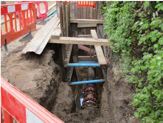
Second Excavation extended for pipe insertion
