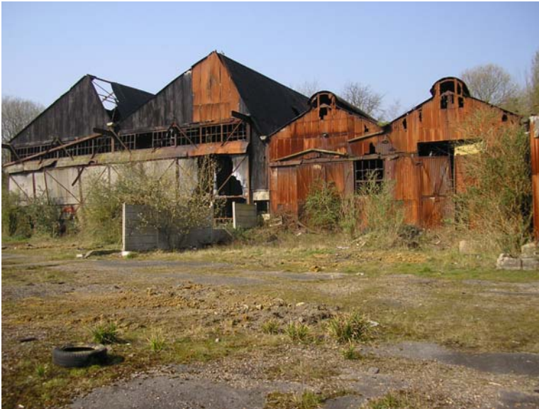
Old Service bay is on the extreme right of this picture
