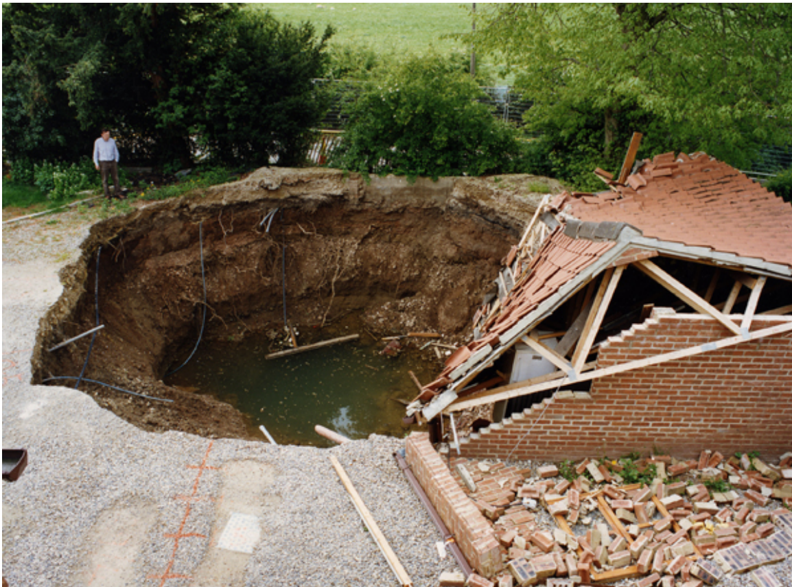
Collapse of four garages into subsidence hollow caused by the dissolution of gypsum at Ripon, North Yorkshire, 1997.
